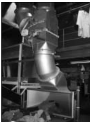
Dryer Vacuum System – Vacuum system carries garments to the dryers which are on a mezzanine above the washers.
