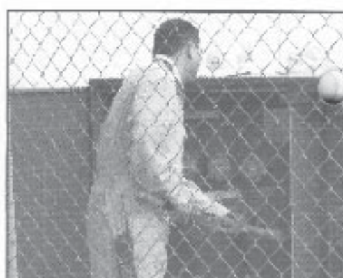
The power company working on the problem.
