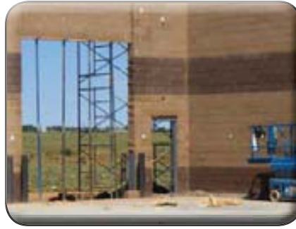
Inside of northwest wall
