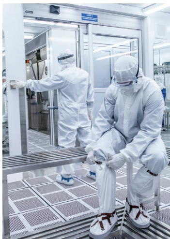
Cleanroom design (including components such as "touch-less" doors and electro-polished stainless steel) as well as proper gowning and operational protocol all play a role in establishing and maintaining an ISO Class 3 (FED-STD-209 Class 1) environment. Pictured is a PCS gowning room.
